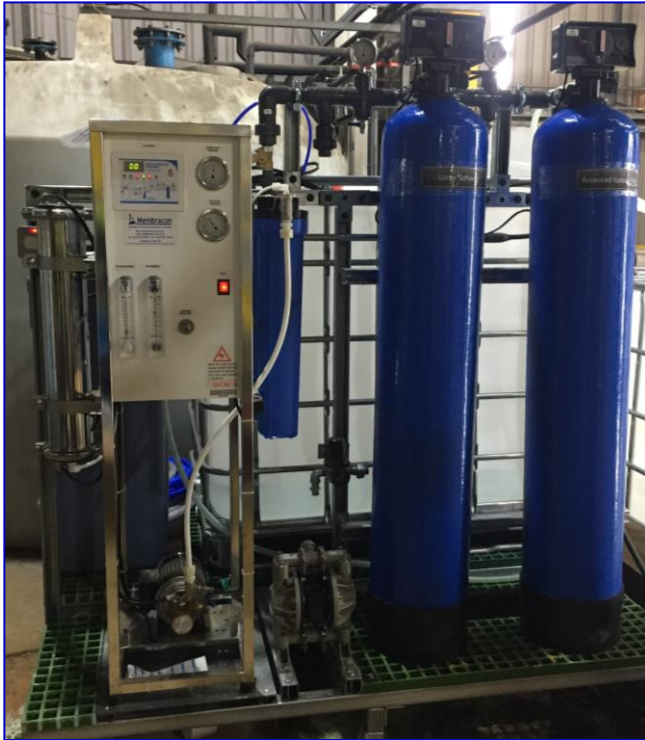
150 lph RO Unit
