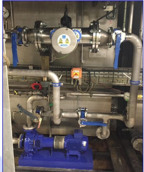
UV Bacterial Prevention System Installed on-site
