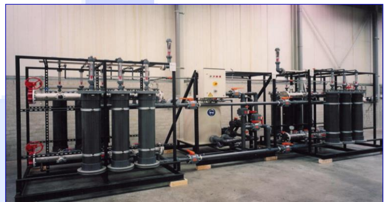
8" UF Rig Including Clean In Place System (CIP). 10,000 ltr/hr Permeate For Automotive & Aerospace Industry
