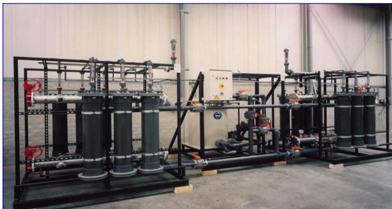
8" UF RIG INCLUDING CLEAN IN PLACE SYSTEM 10,000ltr/hr PERMEATE FOR AUTOMOTIVE & AEROSPACE INDUSTRY
