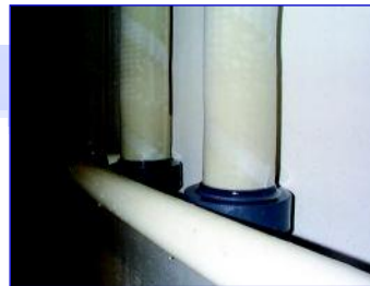
Bumpers to reduce movement behind a crash rail
