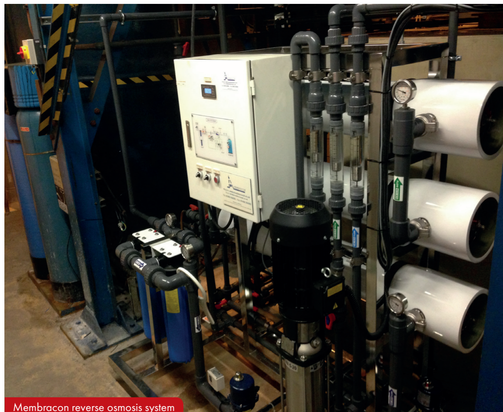
Membracon reverse osmosis system
